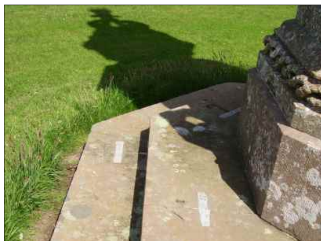
Fig. 2. One corner of the octagonal sundial plinth points north. When the shadow of the obelisk falls on this corner it is local apparent noon. This photograph was taken in the early afternoon when the shadow had moved past the noon point.
