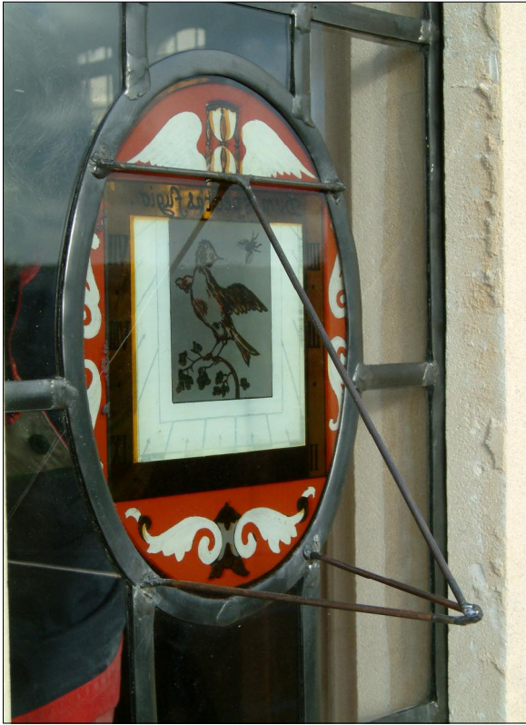
Fig. 4. The dial viewed from outside the building, showing the gnomon supports. The colours look quite different from this side.
