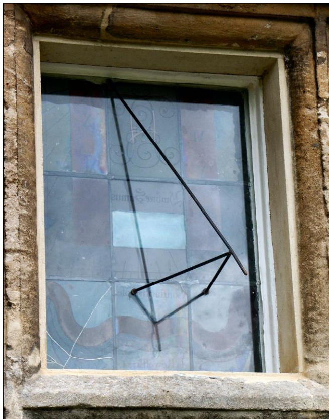
Fig. 12. The replacement gnomon attached to the outer, protective glass sheet.
