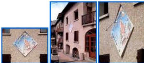
Sundial with Saint Crepin 05, format 120 X 120 cm. A finishing was made to rectify the support of the sundial, the wall not being vertical.
