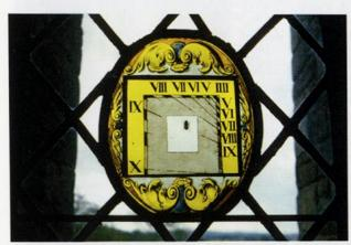
the glass-painter. The dials are calculated and delineated in exactly the same way as for ordinary vertical dials, direct or declining, except that they are made of glass and built into a suitably situated window. The gnomon is fitted on the outside of the window, but the numerals are reversed and read from the inside, so that the viewer need not leave the comfort of the room on a sunny but cold winter's day.
